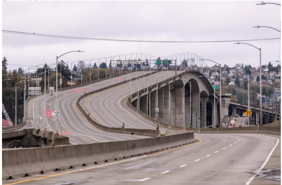
Figure 1: The West Seattle High Bridge (closed to traffic) and the Spokane Street Swing Bridge
