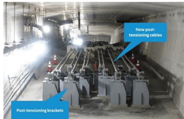
Figure 4: Newly installed post-tensioning cables and brackets in the high bridge
