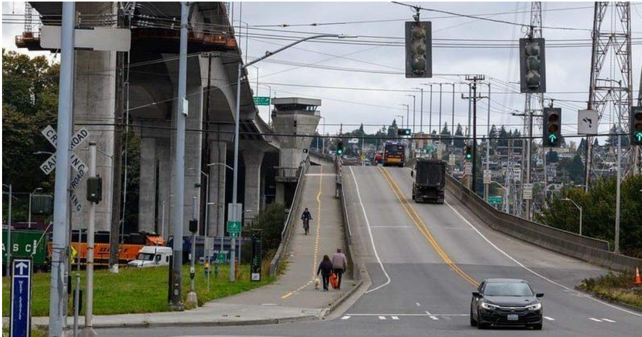
Figure 3: Pedestrians, cyclists, transit, and permitted vehicles may use the Spokane Street Swing Bridge.
